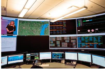
System operators use a curved videowall driven by an Extron Quantum Ultra processor to monitor and manage the public power grid for the state and its service territories. The videowall presents content selected from various video sources, broadcast feeds, and computergenerated graphics and other data in windows of varying sizes and orientations.
