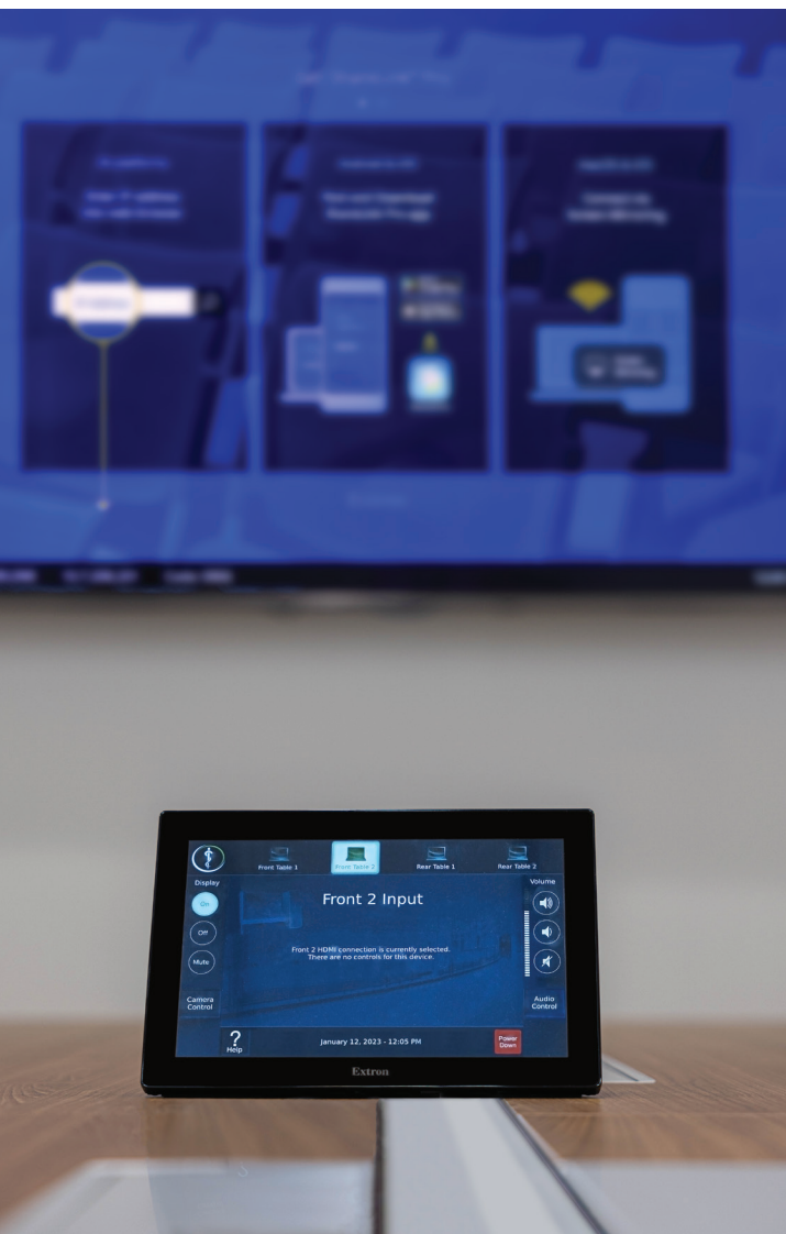
Two conference rooms equipped for Bring Your Own Meeting – BYOM and wireless presentation controlled via Extron TLP Pro 1025T 10" Touchpanel
