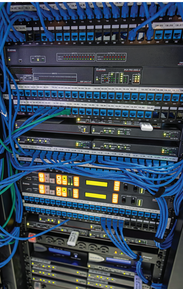
Main AV rack in building two ties all the solutions together with Extron NAV encoders and decoders, NAVigator with 96 Endpoints Upgrade LinkLicense, wireless presentation, streaming and recording, as well as audio and control.
