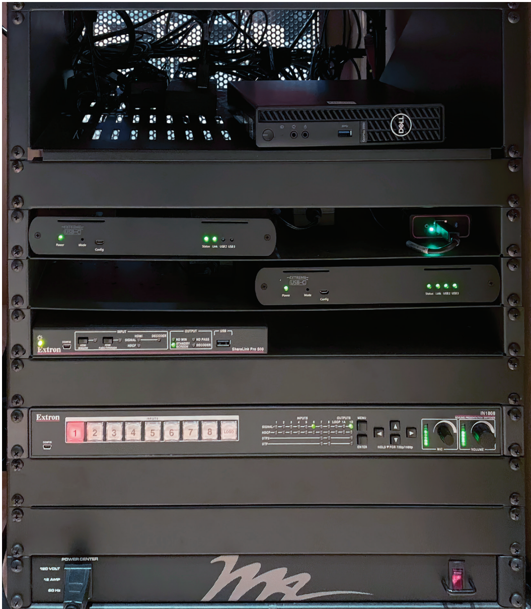
Lectern AV rack with ShareLink Pro 500 presentation gateway and IN1808 scaling presentation switcher.
