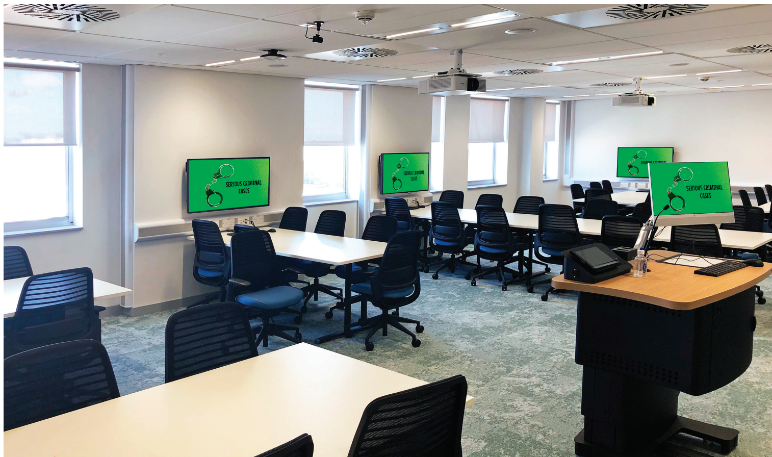
In UWE's collaborative learning spaces, the projection systems are fed by an Extron IN1608 xi scaling presentation switcher. The pod displays follow the main display until a student in that pod selects a different source. Sessions held in the interview rooms are shared live with the classrooms over the NAV® Pro AVoIP system.
