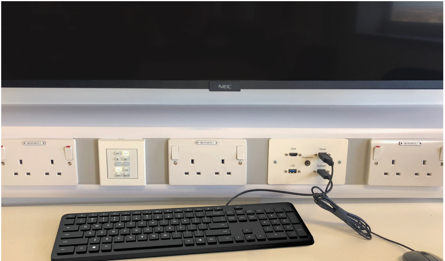
Each of the 18 student pods provides AV connectivity for a keyboard, a mouse, and mobile devices, as well as source switching plus local display control using an Extron EBP 110 MK eBUS® 10-button panel.
