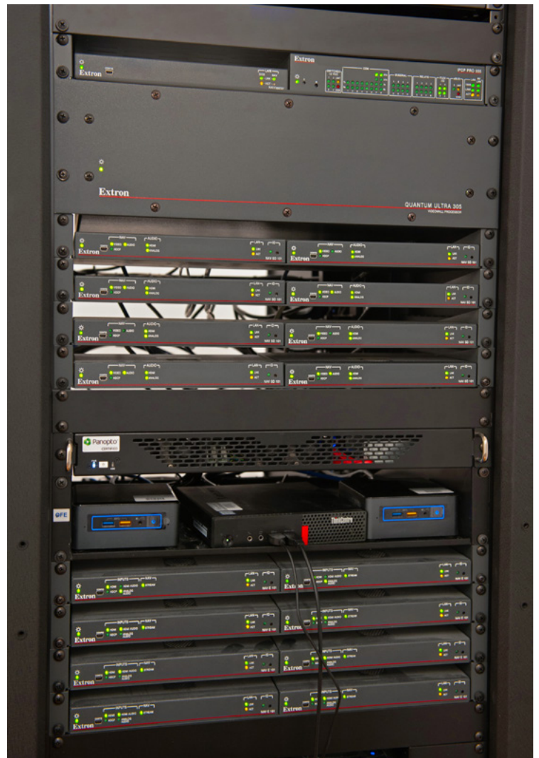
The Control Room rack contains NAV Pro encoders, decoders, and NAVigator, as well as the Quantum Ultra videowall processor, IPCP Pro control processor, and various AV content sources.
