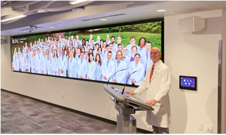
The AV system and room lighting are controlled at the wall-mounted TouchLink Pro touchpanel. Presenters advance and annotate their slides at the smart lectern. Photo courtesy of Heidi Grassley, ClarkPowell.
