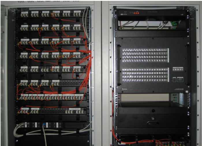
AV equipment vital to AMS operations is rack-mounted in the RAM center.
