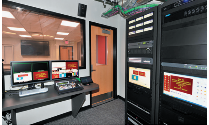
Technicians in the control room can monitor the lecture content recording and assist instructors in operating the classroom's AV system, such as switching between content display configurations.
