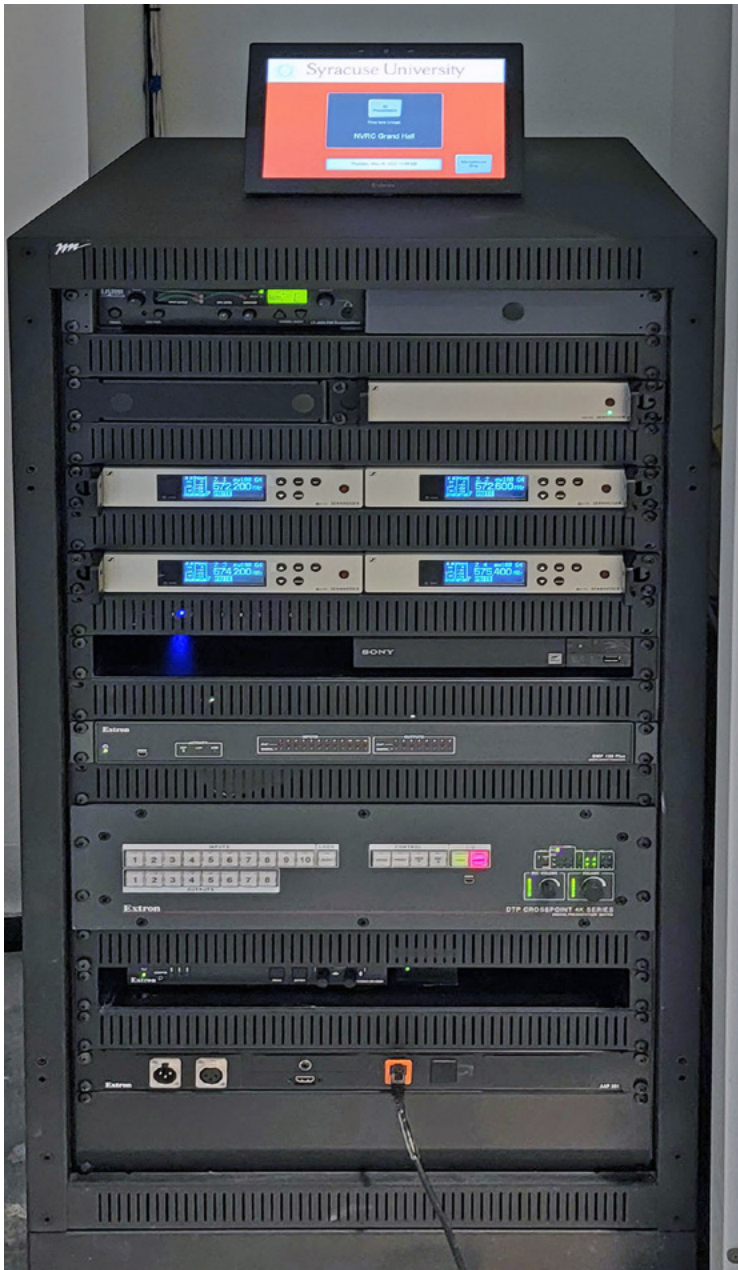
In the Grand Hall, the AV products are rack-mounted in an equipment room. An Extron TLP Pro 1025T 10" TouchLink Pro Touchpanel on the rack offers local system control.
