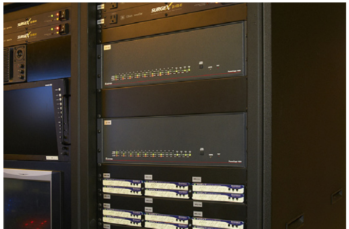
The Extron PowerCage 1600 enclosure simplifies integration for large fiber optic systems, providing a convenient way to rack mount multiple transmitters and receivers.
