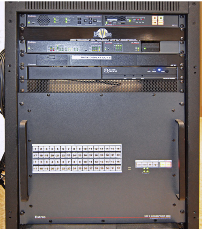
The XTP II CrossPoint 3200 matrix switcher and other system components are rack-mounted in the adjacent equipment room. This space is also used to store spare gaming gear and provides a small work space with a connected monitor.
