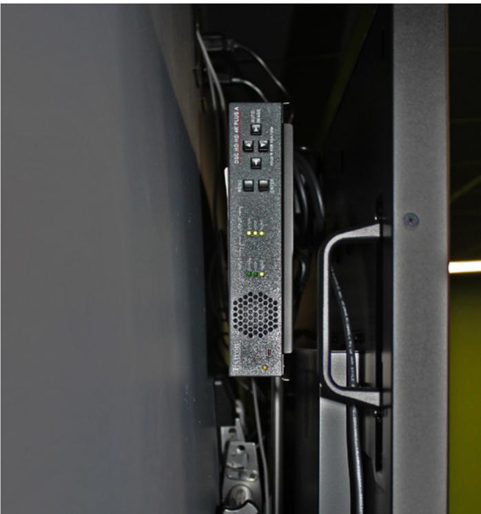
The DSC HD-HD 4K PLUS A mounted behind each wall display scales the 2560x1440 signal from the gaming PC to the display's native resolution. The scaler for the center display also de-embeds audio to support the sound system.
