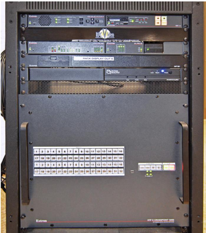
The XTP II CrossPoint 3200 matrix switcher and other system components are rack-mounted in the adjacent equipment room. This space is also used to store spare gaming gear and provides a small work space with a connected monitor.
