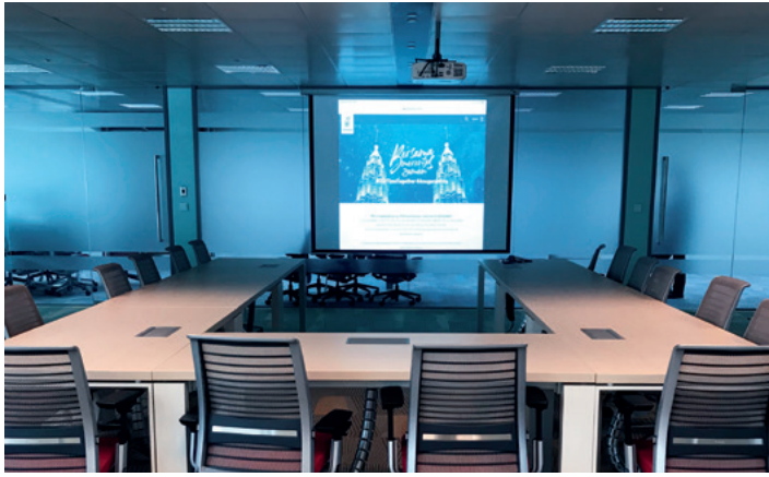
Typical conference room AV collaboration system setup at Petronas headquarters includes one or more Cable Cubby enclosures, a switching transmitter and scaling receiver pair, and a ceiling-mounted projector.
