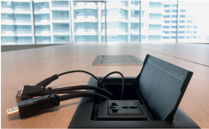
Seen in this view from a meeting room in one of the Petronas twin towers, a Cable Cubby 202 cable access enclosure provides meeting participants with a choice of input device connectivity options as well as device power. A cable retractor allows users to extend cables to connect to their devices and pulls cables back into the enclosure when not in use.
