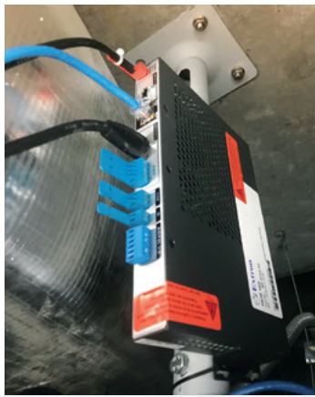
The HC 404 switching transmitter mounted beneath the conference table (left) extends user audio, video, and control to the ceiling-mounted projector located up to 230 feet (70 meters) away over CATx cable via an HC 404 scaling receiver mounted above the ceiling (right). Also shown on the left is a cable retractor installed beneath the table.
