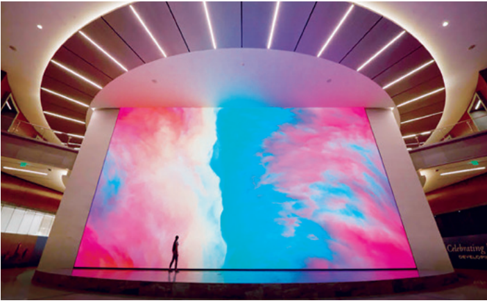
Genero outfitted the vast lobby with a NanoLumens 4 mm direct view LED videowall measuring 36' x 64', which is driven by an Extron Quantum Ultra 610 4K Videowall Processor. By default, custom content produced by Second Story fills the entire canvas. Pictured: Second Story's generative media artwork, Unify. Photo credit: Second Story
