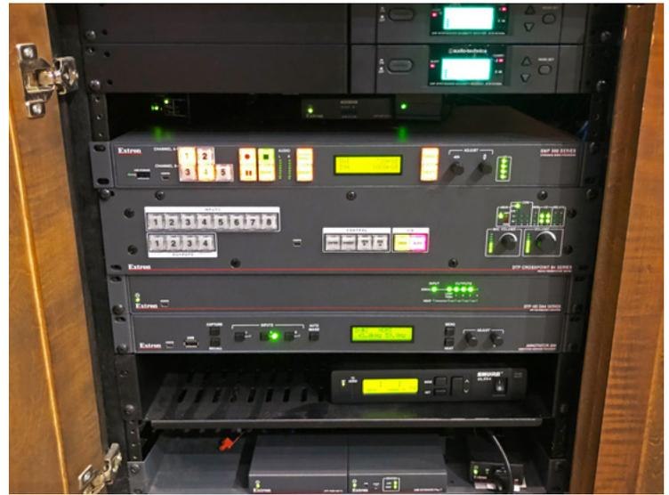
AV Operator desk equipment bay showing some of the Extron components. Top to bottom: SMP 351, DTP CrossPoint 84 4K, DTP HD DA4 4K, Annotator 300. DTP HDMI 4K 230 Tx and USB Extender Plus T are at very bottom.
