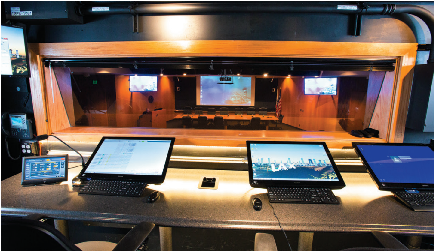
The mezzanine-style control room offers complete AV system operation and a clear view of displayed content within LAX's 100-seat Samuel Greenberg Boardroom.
