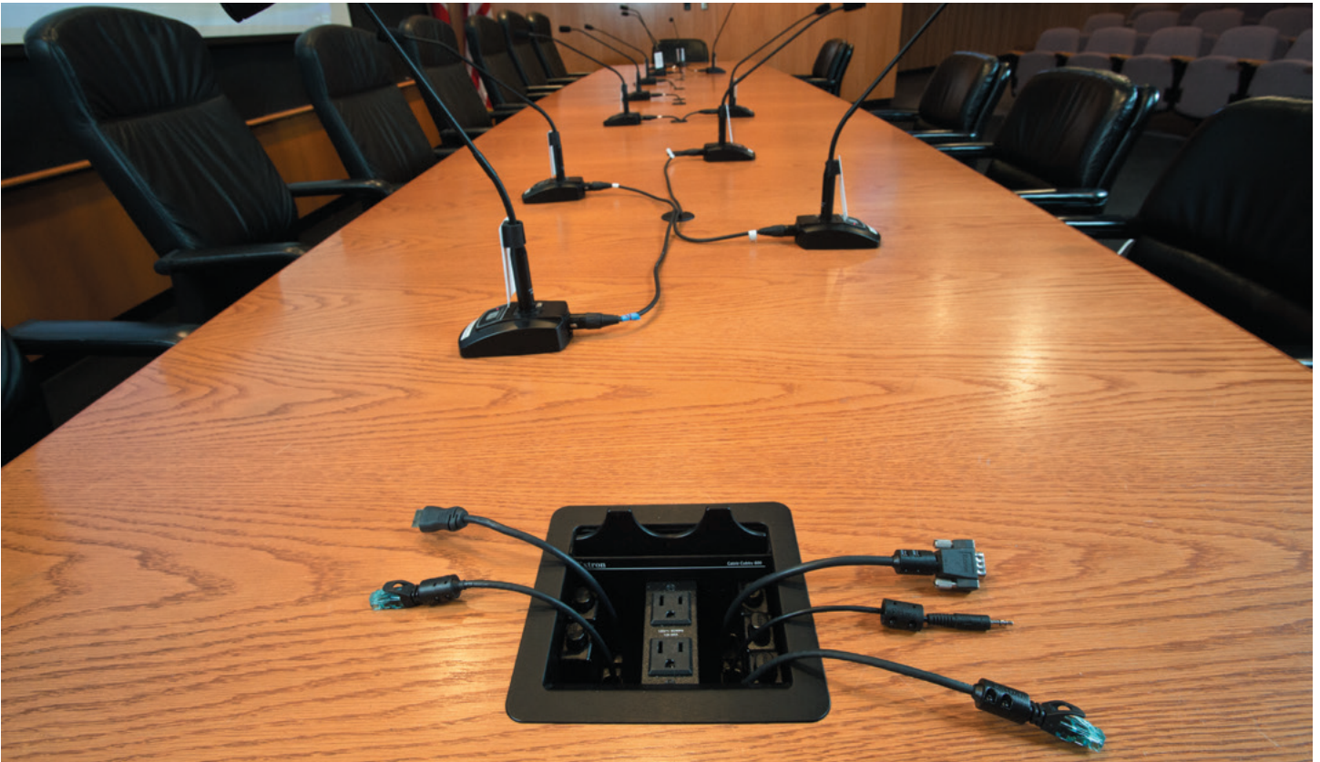
Cable Cubby 600 enclosures installed in the lectern and at both ends of the head table offer HDMI, VGA, Audio, and LAN connectivity plus power for portable devices.
