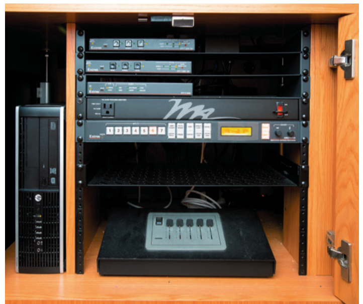
Two XTP T USW 103 switchers and the Annotator offer local or connected source selection and presentation enhancement from the front of the room.
