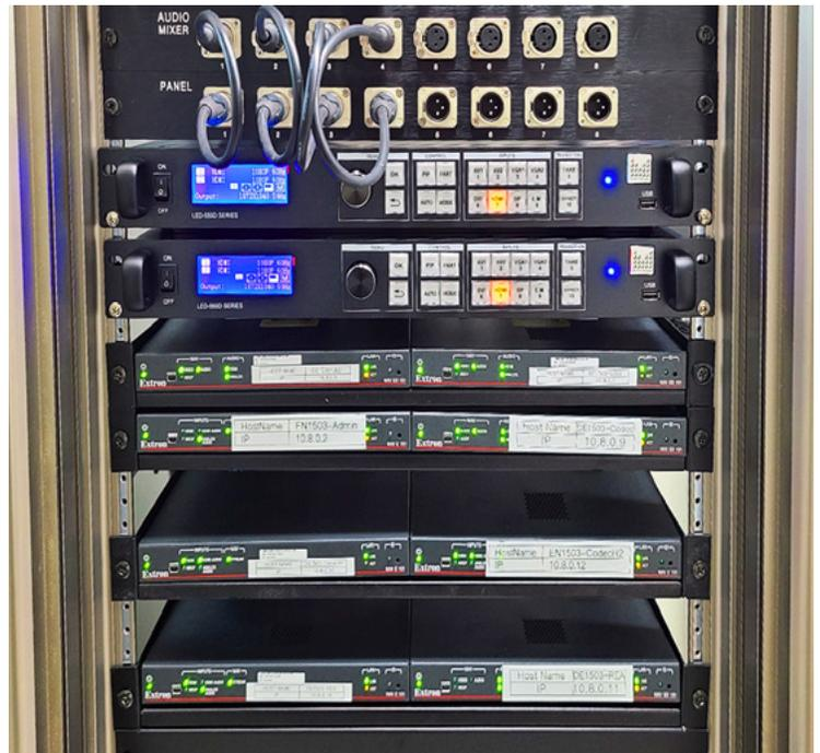
The three conference rooms are each equipped with an AV rack containing four NAV Pro encoders and four decoders that implement the AV over IP network in conjunction with the Ethernet switch at the top of the rack that works with the building's enterprise data network. Photo courtesy of Neuroo Digitech.
