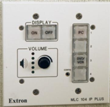
**The MediaLink control panel makes it easy to turn the projector on and off, select inputs and adjust the volume.**
