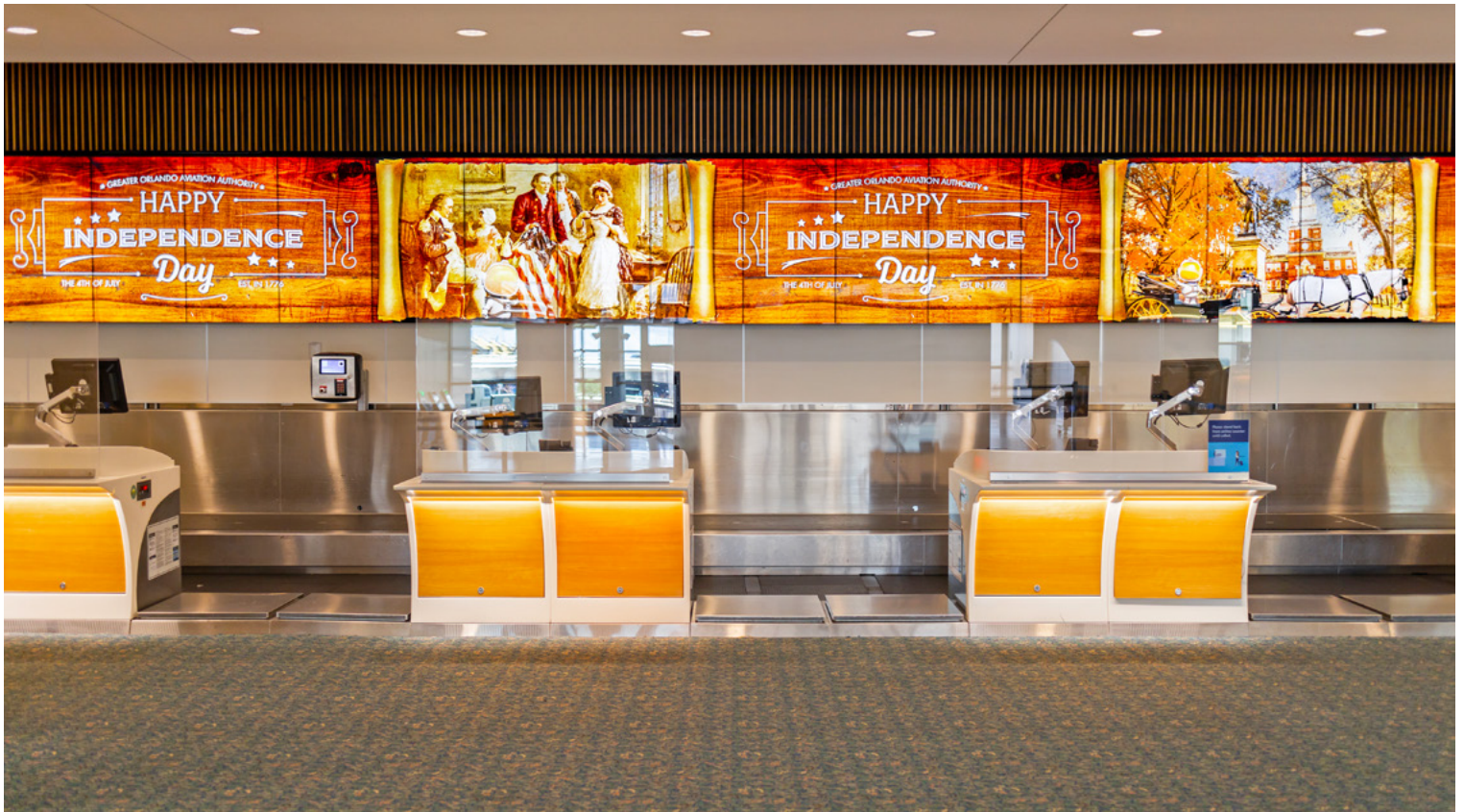
A videowall comprised of 700 synchronized screens creates a seamless canvas running behind the ticketing counters. It provides the flexibility to reassign ticketing counters among the 40 airlines according to demand and shows seasonal messages for unused counters.
