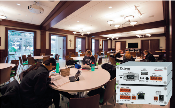
Existing audio systems in some venues, such as the dining facility pictured here, were easily integrated with the GVCCS PA and bell system via CC 100C Codecs (inset).
