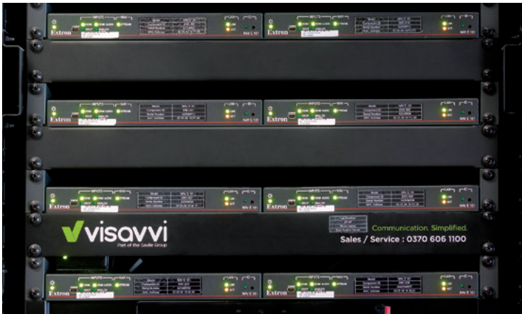
Eight NAV E 101 Pro AV over IP Encoders place 4K HDMI video from eight PCs onto the facility's 1 Gbps Ethernet network. These encoders share rack space with the PCs in the Communications Room.
