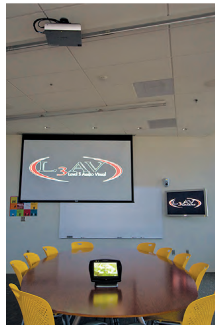
HD videoconference cameras are tied to the central codec farm using MTP series twisted pair transmitters and receivers.
