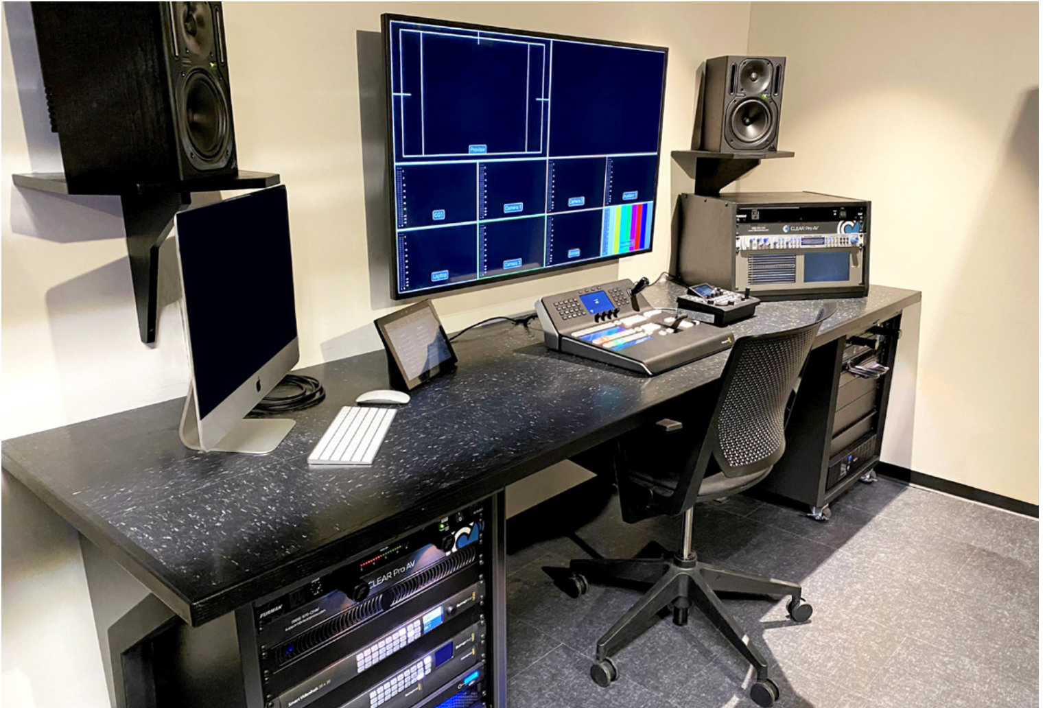
Adjacent to the theater is the control room, facilitating operation of the AV system that functions independently from the Cinemark projection installation. All photographs courtesy of Clear ProAV.
