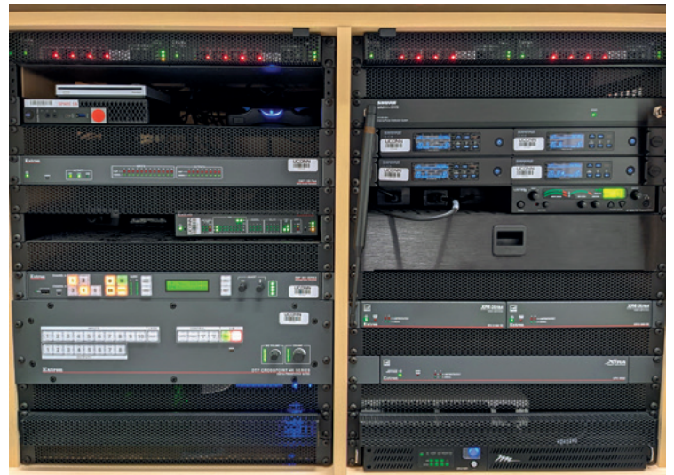
The left side of the Gant lecture hall teaching station houses AV sources, switching, distribution, streaming, and control equipment as well as a digital matrix processor for mixing and processing audio. The right side contains wireless mic receivers and audio amplifiers.
