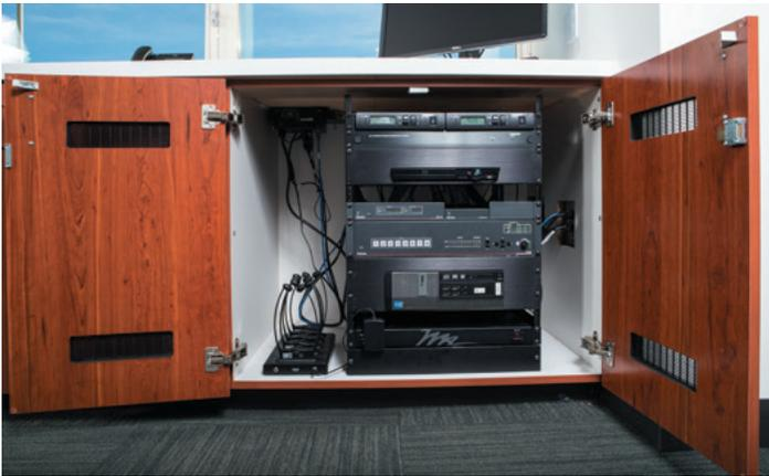
An Extron IN1608 scaling switcher in each Instructional Support room enables easy signal routing from a wide variety of sources.
