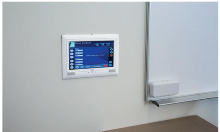
TLP Pro 1020M 10" TouchLink Pro touchpanels are mounted on the front and back walls of each lecture hall, allowing the instructor to move about the room.
