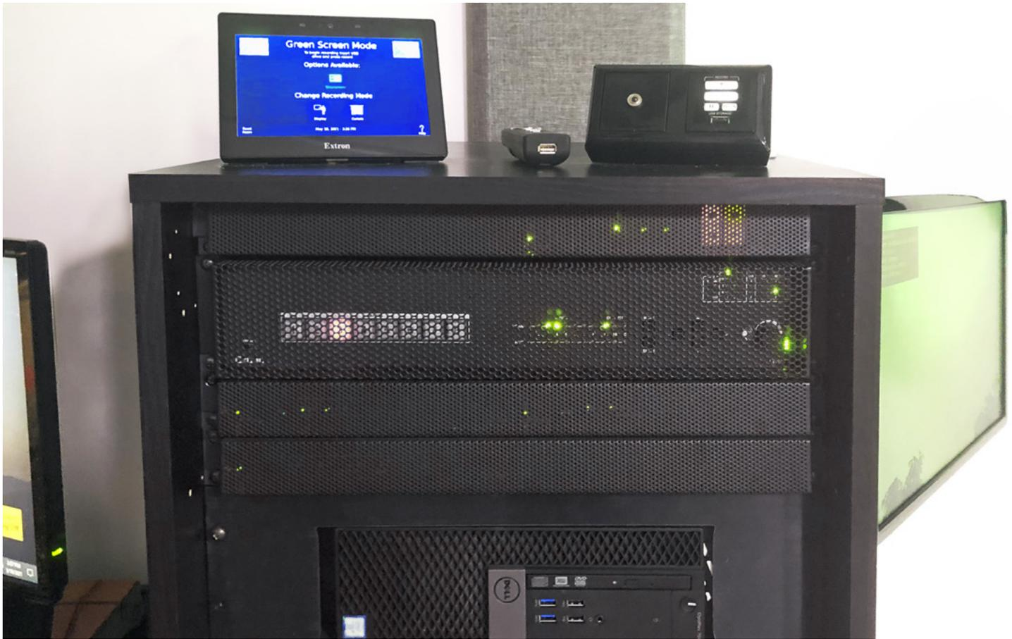
Main AV equipment rack. TLP Pro 725T 7" TouchLink Pro touchpanel, RCP 101 remote control panel, and presenter's remote control are on top of the rack. Visible within the rack are the IN1608 xi scaling presentation switcher and the PC. A confidence monitor swings out from the right side of the rack.
