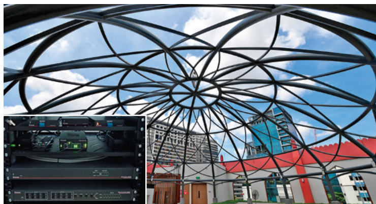
New auditorium and dual-use outdoor communal pavilion topped by a modern lattice dome on the fourth floor. These venues obtain AV content via their own sub-distribution system with dedicated matrix switcher and distribution amplifier (inset).
