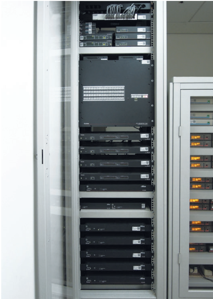
An Extron XTP CrossPoint 3200 modular matrix switcher provides signal routing throughout the 13-way divisible training space on Level 9. Photograph courtesy of PT AIA Financial (AIA).
