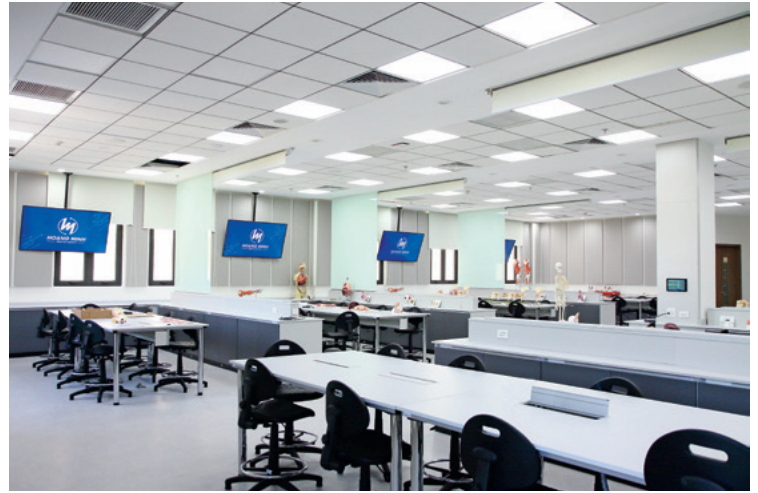
Each display can show different material at resolutions up to 4K/60, with the source content routed by an Extron DXP 168 HD 4K PLUS matrix switcher.
